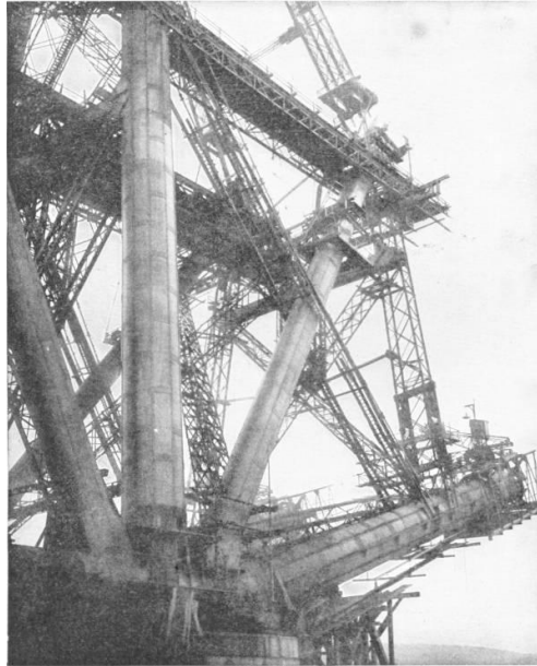
CONSTRUCTIONAL DETAIL OF THE FORTH BRIDGE
